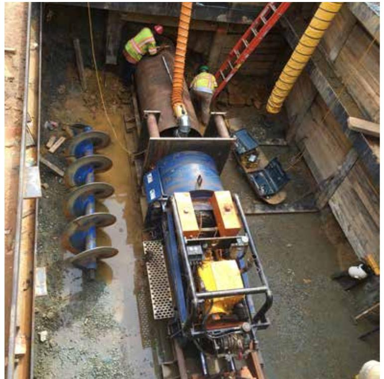
A jack-and-bore process allowed for ductbank installation along a busy street without closing the street to traffic. *Photo: Dewberry*
